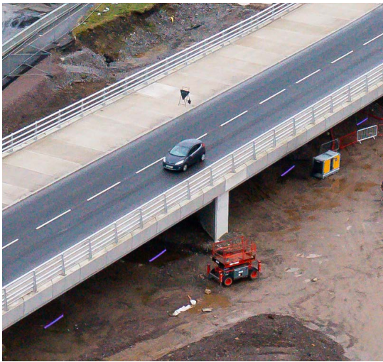
Trewaun West Bridge
