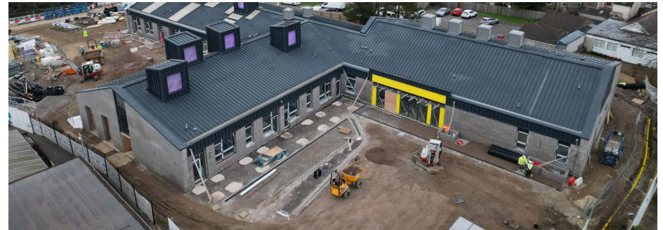
Llanilltud Primary School – drone view
