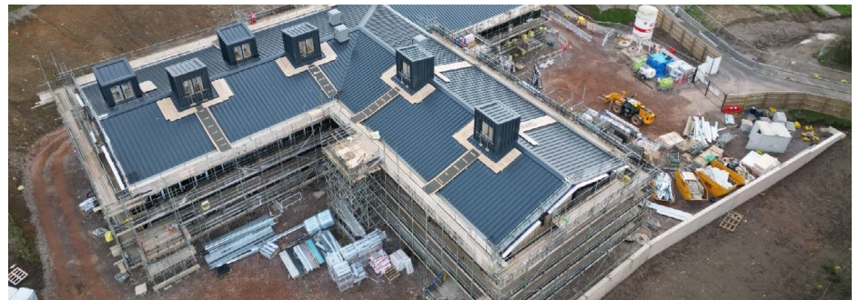
Penygawsi Primary School – drone view
