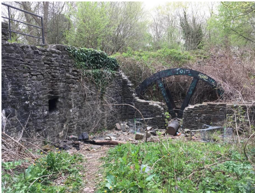
Fig. 1. General view of the remains of the woollen mill (28/04/21)
