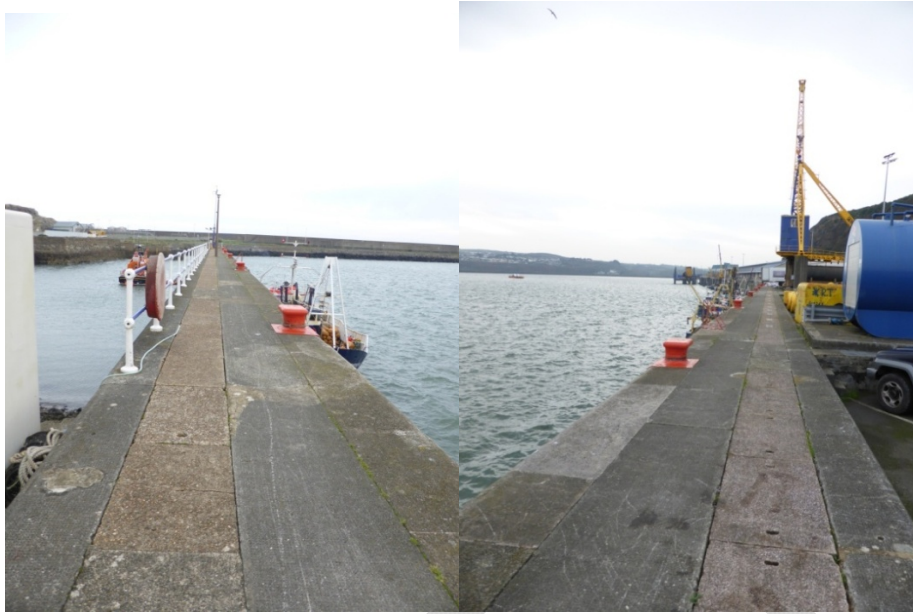
Figure 3.3 & 3.4 Northern Quay, Facing North and Facing South
