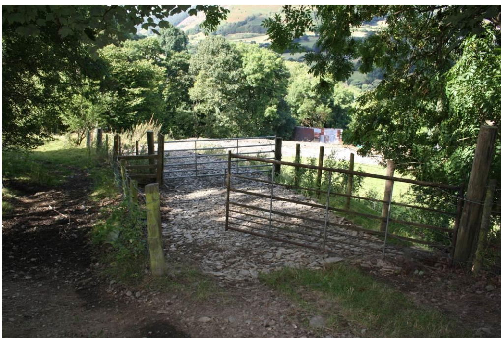
Cadw - DE246 - Deeside Slateworks - 2016-09-08 - 06 - View of new track, facing WNW
