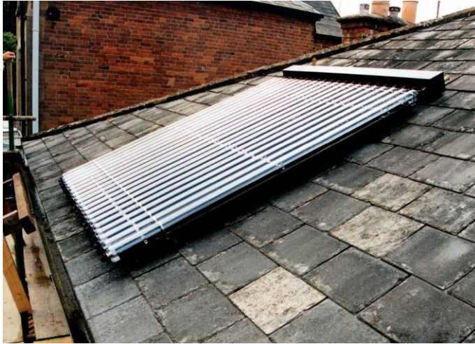
Figure 2.7: Solar thermal panel (evacuated tube system) [Source: www.cse.org.uk ]
