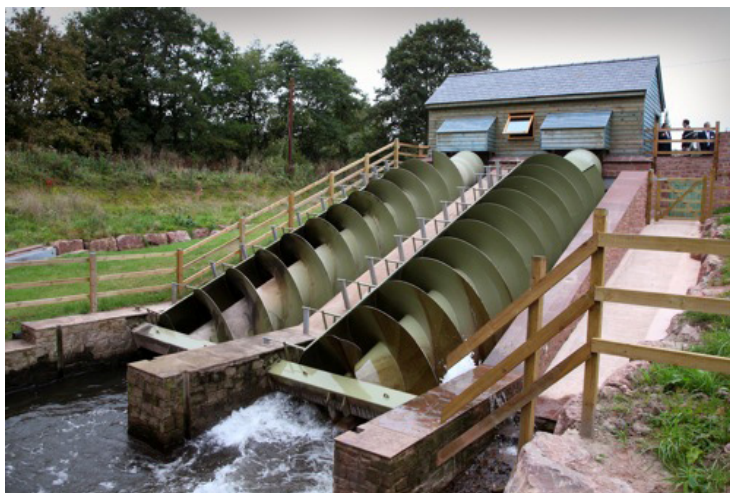
Figure 2.6: Osbaston 150kW hydropower scheme and fish pass on the River Monnow in Monmouthshire, opened 2009. [Source: www.aberdareonline.co.uk ]
