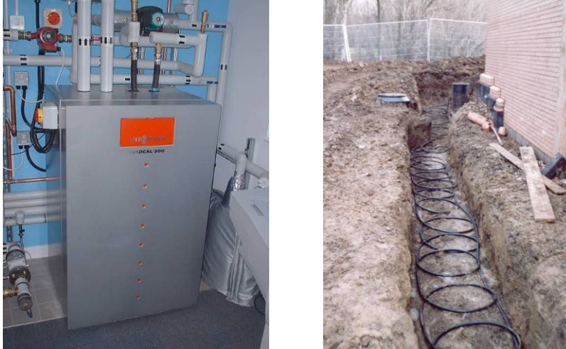
Figure 2.10: Ground source heat pump unit (left) and 'slinky' ground loop (right) [source: www.gshp.org.uk ]
