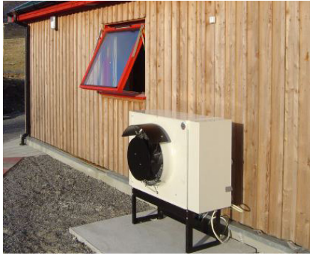
Figure 2.1 I: Air source heat pump unit [source: www.airsource-heatpump.co.uk ]
