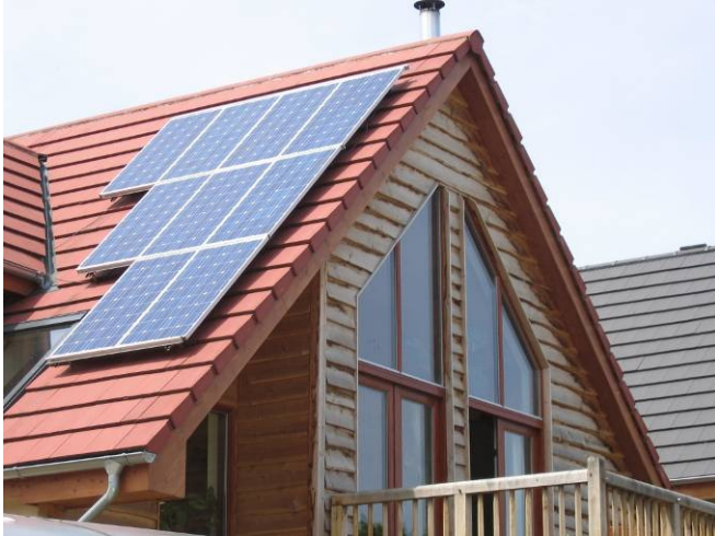
Figure 2.8: Retrofit solar PV panels [Source: www.cse.org.uk ]
