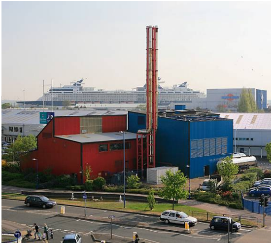
Figure 2.12: Southampton Geothermal plant [© Copyright Peter Facey; licensed for reuse under Creative Commons Licence ]
