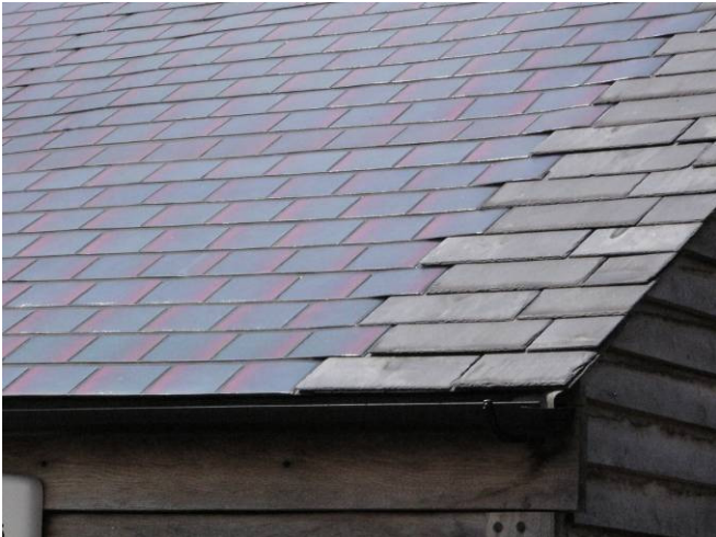
Figure 2.9: Building-integrated solar PV tiles [Source: www.cse.org.uk ]
