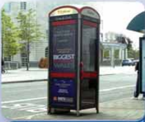
Telephone box houses microcell
