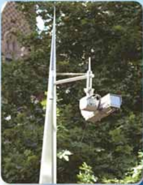
Antenna in combination with local CCTV scheme
