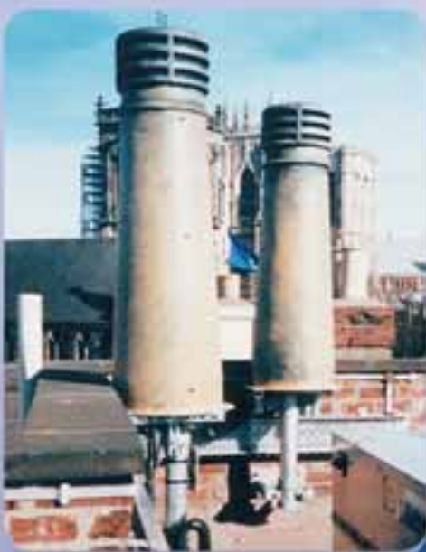
Antenna concealed in GRP chimney pots
