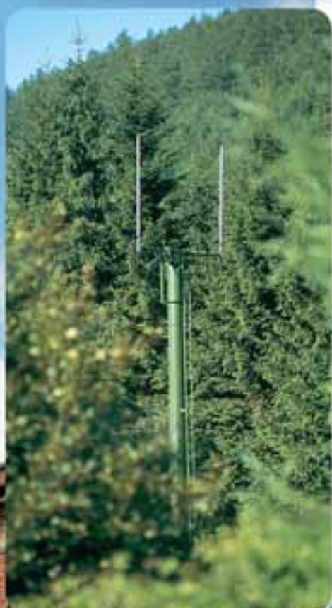
Monopole mast painted green with antennas
