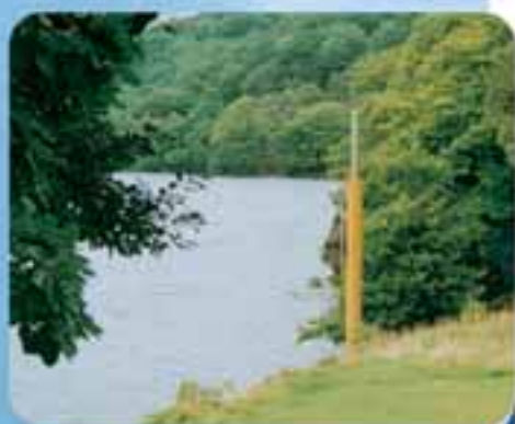
Electricity cable marker used to incorporate antennas
