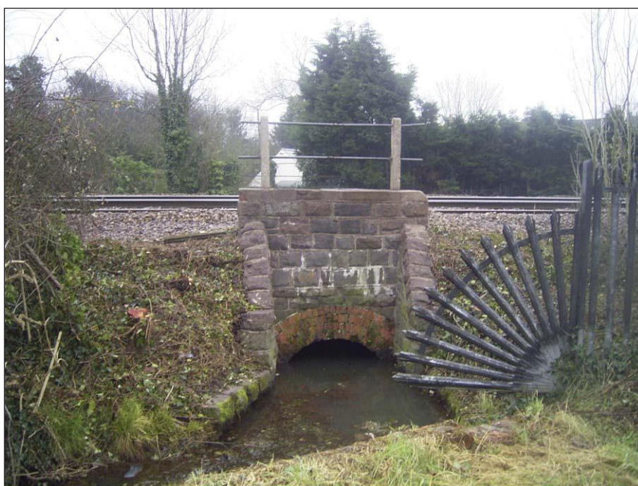
Plate 4: Culvert taking Old Diary Reen under the railway
