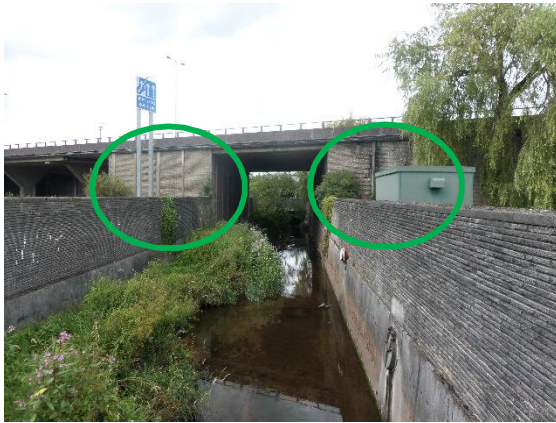
Plate 3: Malpas Viaduct – The central Internal Spaces (Circled in green)
