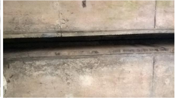
Plate 2: Malpas Viaduct – Expansion Joint
