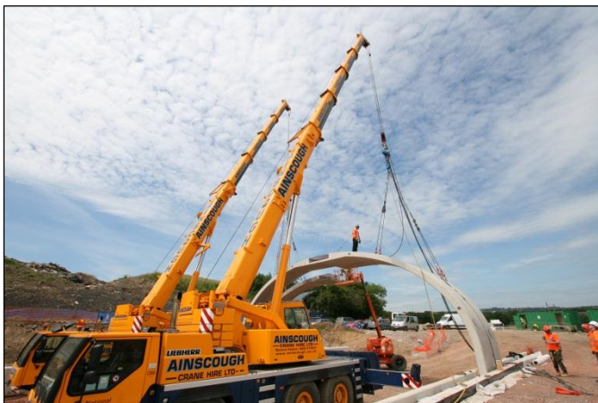
Construction of a precast concrete arch bridge/ Adeiladu pont fwa o goncrïd wedi'i rag-gastio
