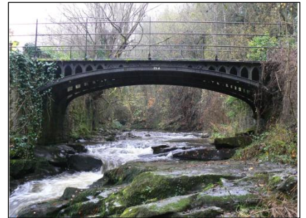
Smart's Bridge/ Pont Smart
