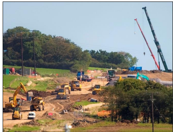
Earthworks Operations/ Gweithrediadau cloddio tir
