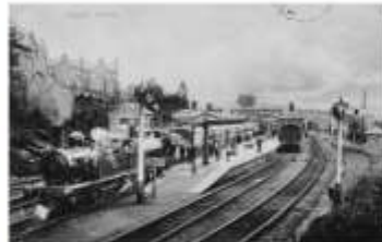
Original "Refresh" is the far structure, also original footbridge which we plan to rebuild. This also shows the Island Platform being used much as we propose.
