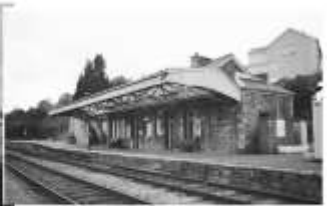
ORIGINAL "Refresh" just before it was demolished without warning by BR in the 60s. It is much missed.
